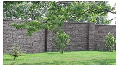
Demonstration walls from five different manufacturers have been constructed to provide the public with an opportunity to comment on which features of the walls they find appealing. Nearly 1.5 miles of sound wall will be constructed at this location in 2008 to help reduce the impact of traffic noise on the Maplebrook neighborhoods.
